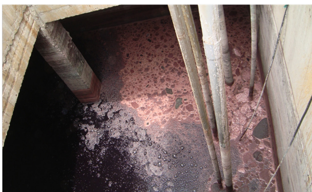
Figure 1. Equalization Tank (capacity 2250m 3 ) of the ETP of Echotex Ltd Chandra, Gazipur, Bangladesh
