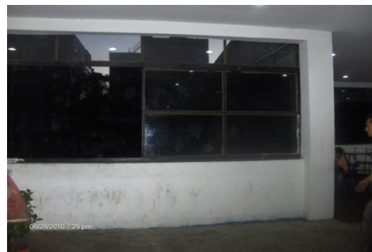
Figure 1. Partially infilled framed structure
