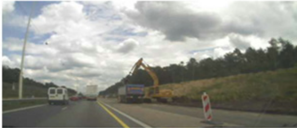
Current Road works (A28)
