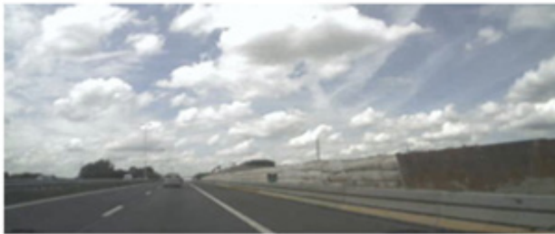
New Road works (A12)
