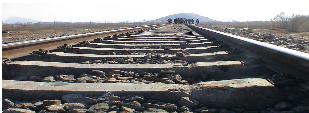
Figure 3. Sleeper breakage due to derailment
