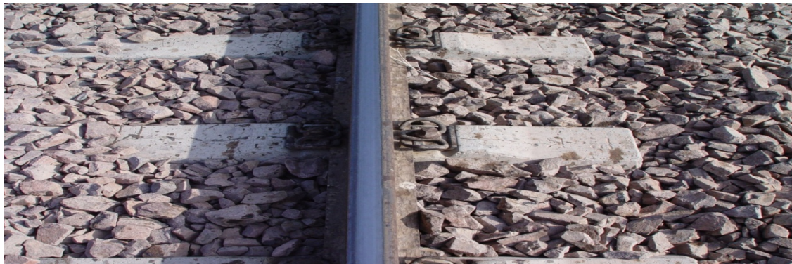
Figure 2. Longitudinal crack in concrete sleeper
