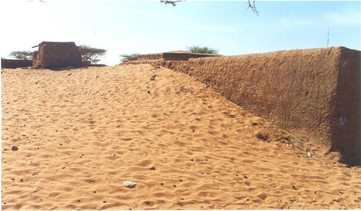
Figure 4. The impact of desertification (moving sand), on houses in Nile state, Sudan (Photo: Mohamed El Fadl)
