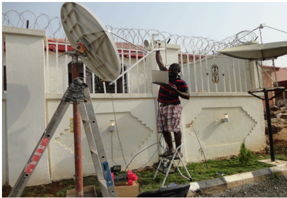
Figure 15. Deployment of 1.2m VSAT Antenna using NIGCOMSAT-1R Satellite
