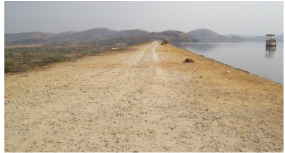
Plate 1. The Lower Usuma Dam Crest
