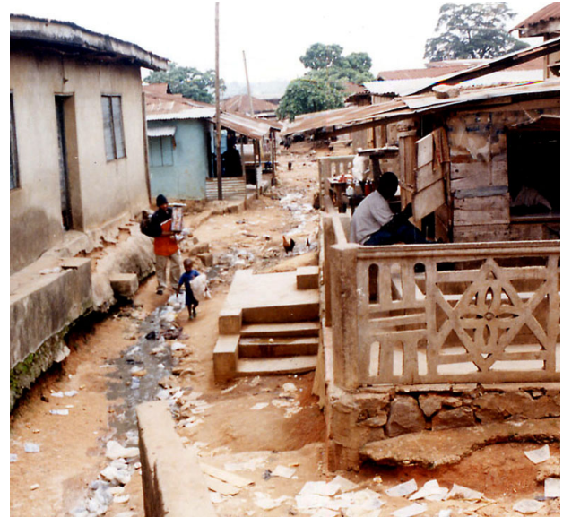
Plate 2. Cement houses opposite makeshift wooden houses in Ojoo, Ibadan. Source:[7]
