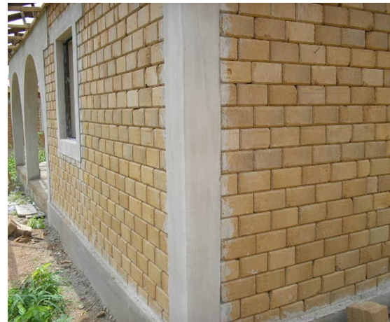
Figure 3. Interlocking Masonry at the finishing stage of a housing project
