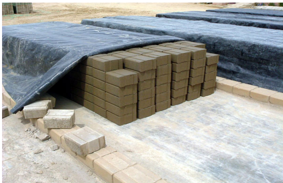
Figure 2. Stacking of Solid Interlocking blocks in a project site
