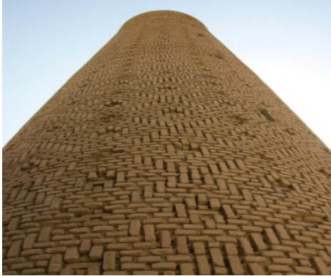
Figure 4. The Barsian Minaret brick work
