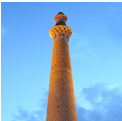
Figure 8. The Sareban Minaret view
