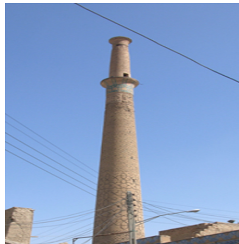
Figure 7. The Ali Minaret elevation
