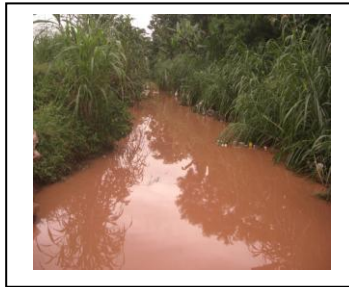
Figure 8b. Drainage route at Works Layout Area, Owerri photographed on 6 th October 2011
